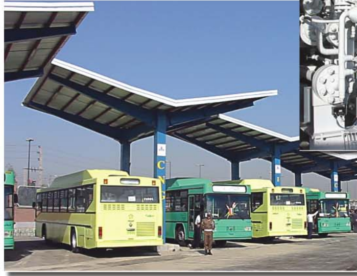
UBCT bus station Site: Teheran, Iran LMF CNG compressors with 2 BS 302-313 S 25
